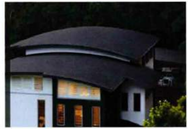
Steel curve roof
