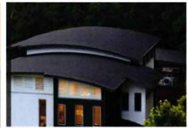
Steel curve roof
